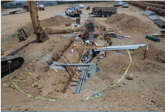
MOH GYM ELECTRICAL
